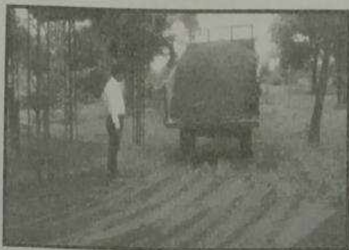
Photograph 4: Leveling of premises of Cremation place by murrum near main road Tundri
