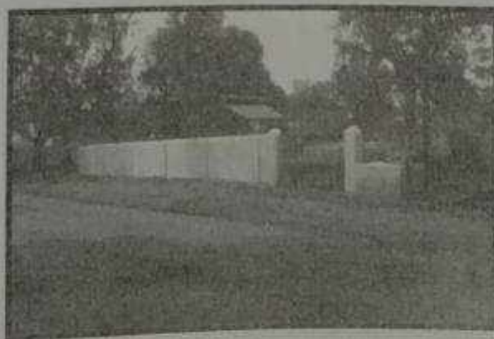
Photograph 36: Cleaning & Painting of cremation shed at Tundri
