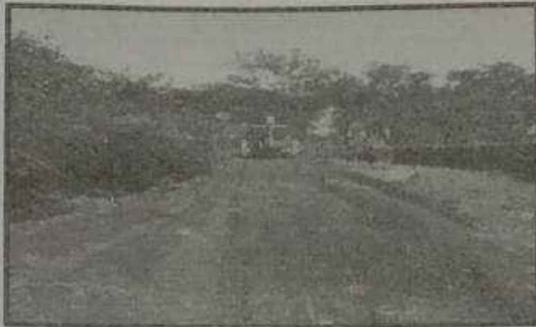
Photograph 6: Village Road Repaired by Murrum at Badadarha
