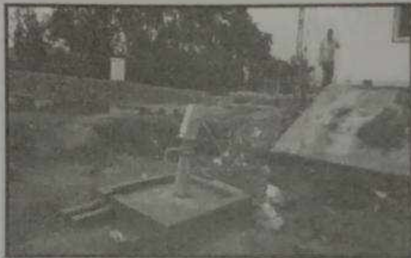
Photograph 3: Installation of Hand pump near LC
