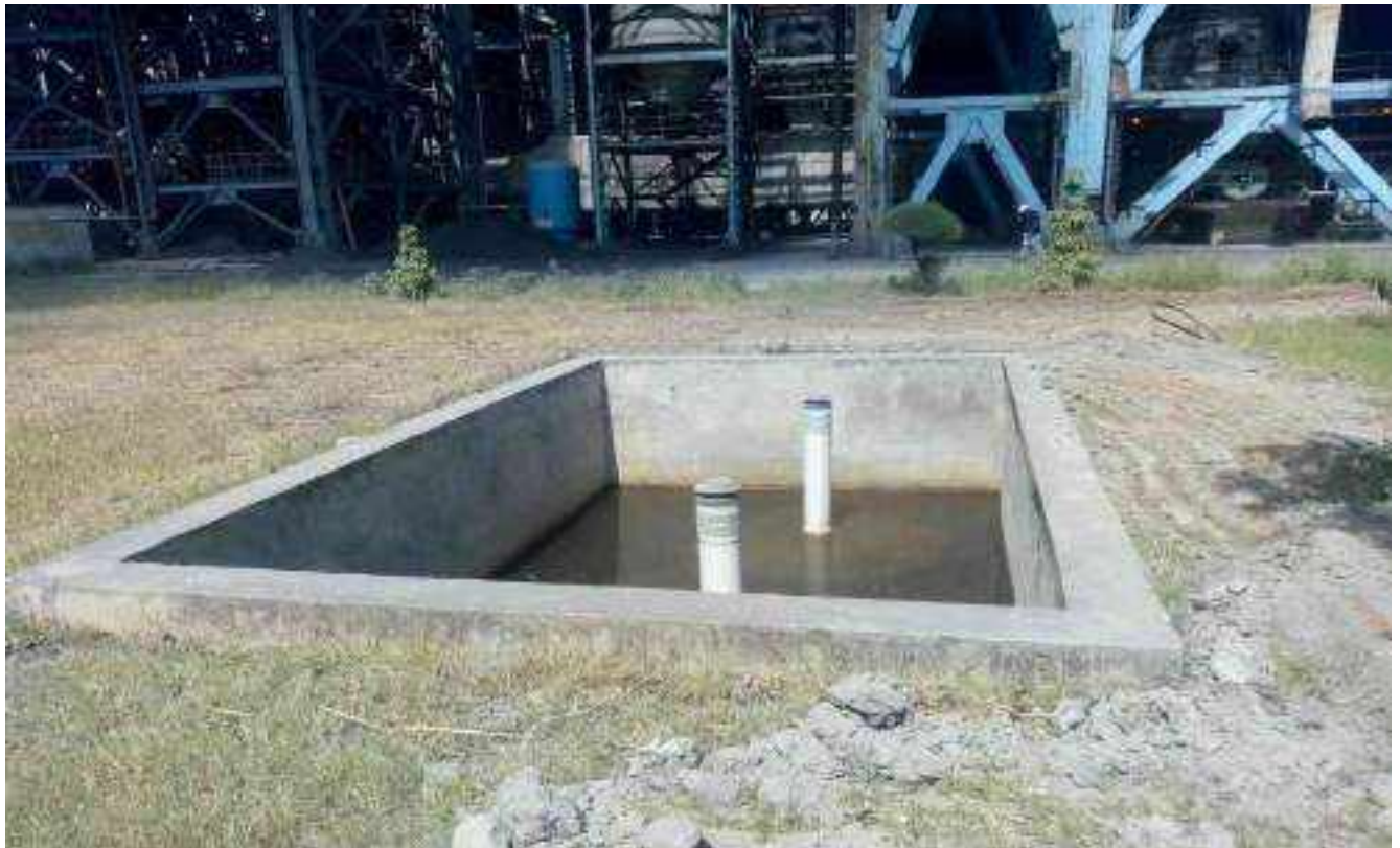
Fig 7.1: Rain water Harvesting in the plant premises
