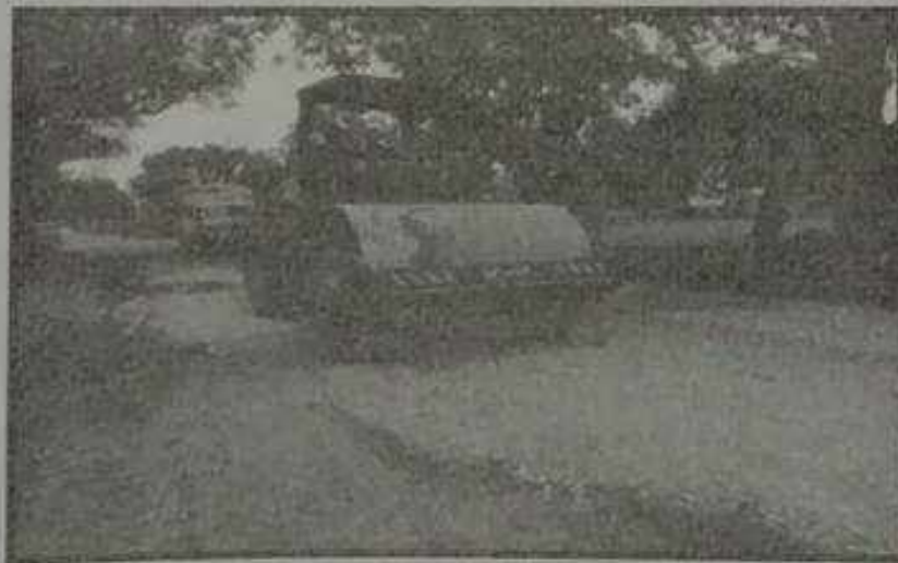
Photograph 7: Repairing of main road
